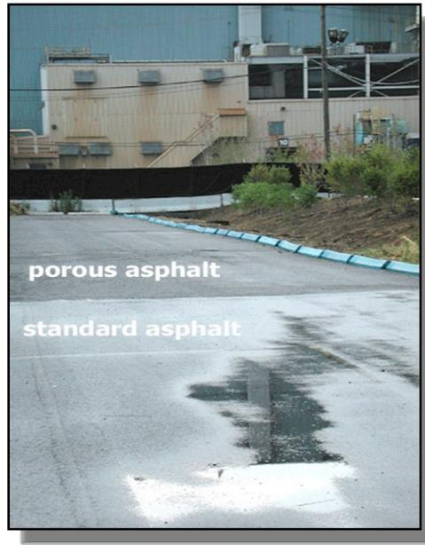
This direct absorption will prevent icing on pathways. Permeable pavements could be used anywhere conventional pavement is used. However, permeable concrete surfaces should not be used for roadways larger than local or residential roads due to traffic frequency.
